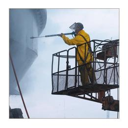
PFX21-08 - A new development by Parker Hannifin in DN12 with 2100 bar working pressure - designed for the water blast market. The new design of PFX21-08 offers robustness and long service life designed for the water blast market in accordance with ISO23384, designation B-210/12,5/210 MPa and DIN EN 1829-2.
